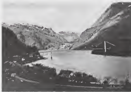
Hardanger Fjord and the bridge at Fykse Sound, Nor.
